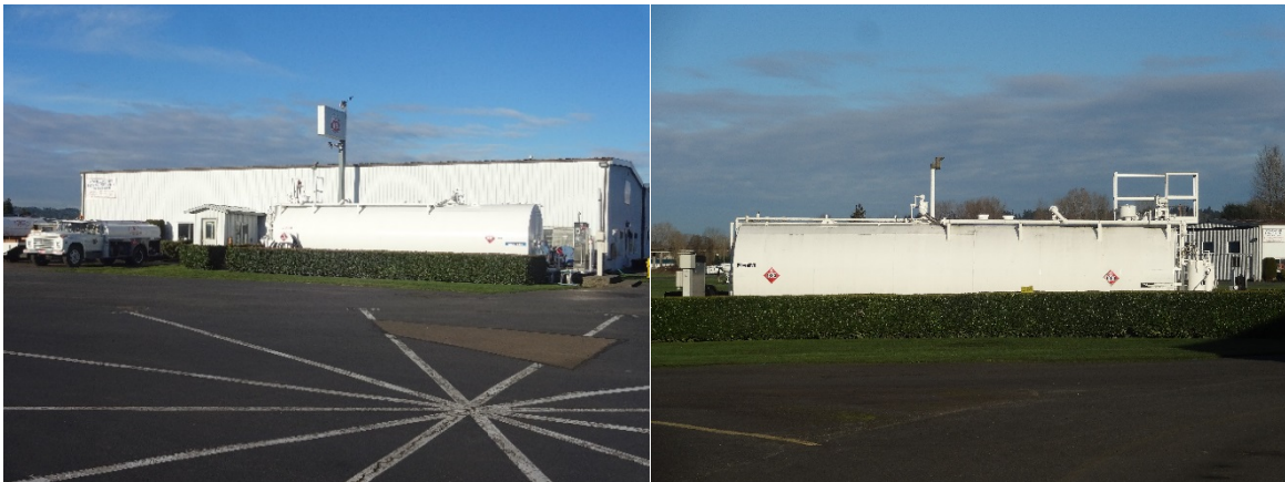
FIGURE 2-15 – S43 AVGAS (LEFT) AND JET A (RIGHT) SELF-SERVE 24-HOUR CARD LOCK
